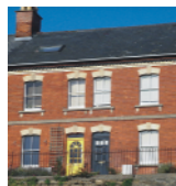
Acquired two storey dwellings Late Victorian to- 1930s - 0.25 to 0.35
